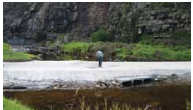
Figure 23 Fish way on Cumberland River Estuary
