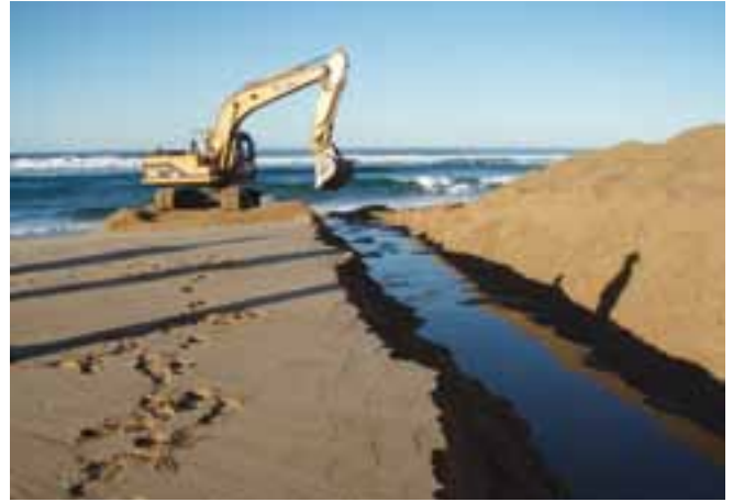
Figure 25 Artificial estuary opening
