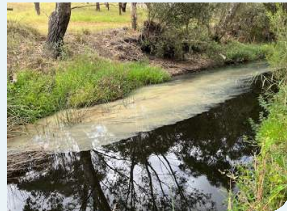
Ooze from a pipe
