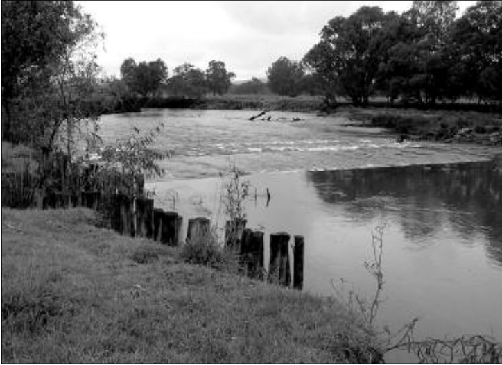
Timber pile fields rectify an unnatural flow split between Murray River and Dights Creek
