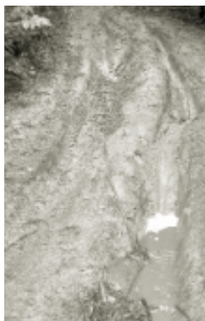
4WD track erosion picked up by turbidity event monitoring on Mortimer Creek.
